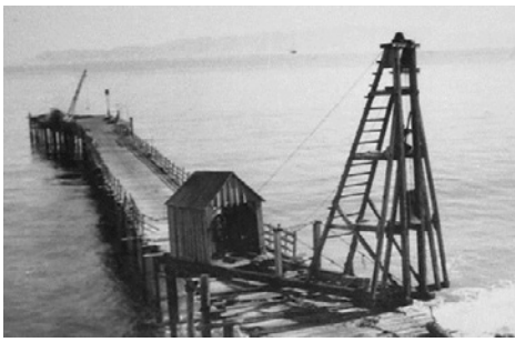
The pier with pile driver in operation.
