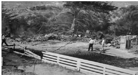
The ruins of the foreman's house and bunkhouse following the fire of 1969.
